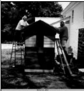
Bob Freitag and Bruce Norton hard at work reassembling the historic
