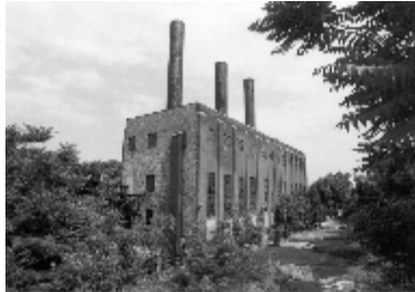
The Beech Street Steam Plant, located within the park, once heated businesses in downtown Akron.
